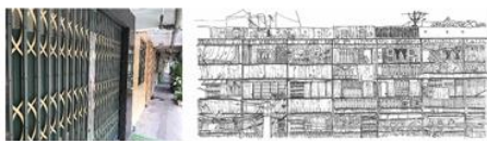
Figure 6. (Left) Front wall of this flat has been replaced with steel sliding panels and granite cladding, (Right) Recording of Chung Cu's facade at present-day (Photographed and sketched by the authors, 2016).
