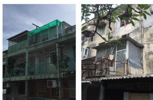
Figure 7. (Left) New structures at Block A, created a fifth level, (Right) Additional 'room' at Block C (Photographed by the authors, 2018).
